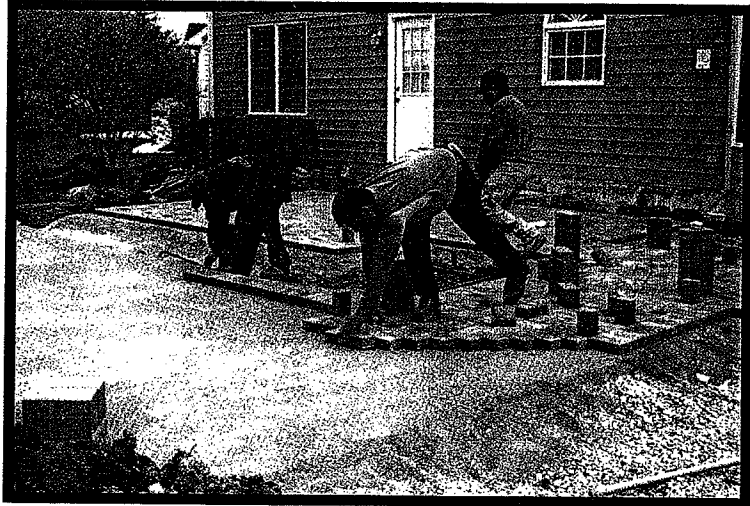
1-20 . These employees demonstrate teamwork in the construction of a patio.
